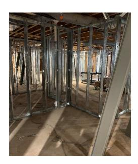
Picture 3: (Red) Assessment wing wall showing the beginnings of rough plumbing installation.
